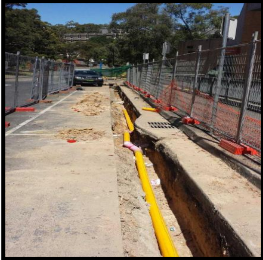
Installation of 250m Nylon Private Main At Macquarie University
