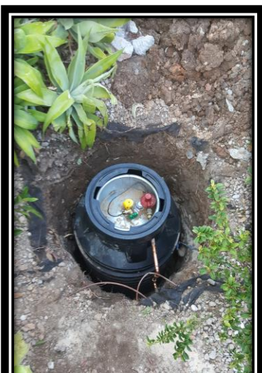
Downunder installation bottle replacement by our Plumbing dept.
